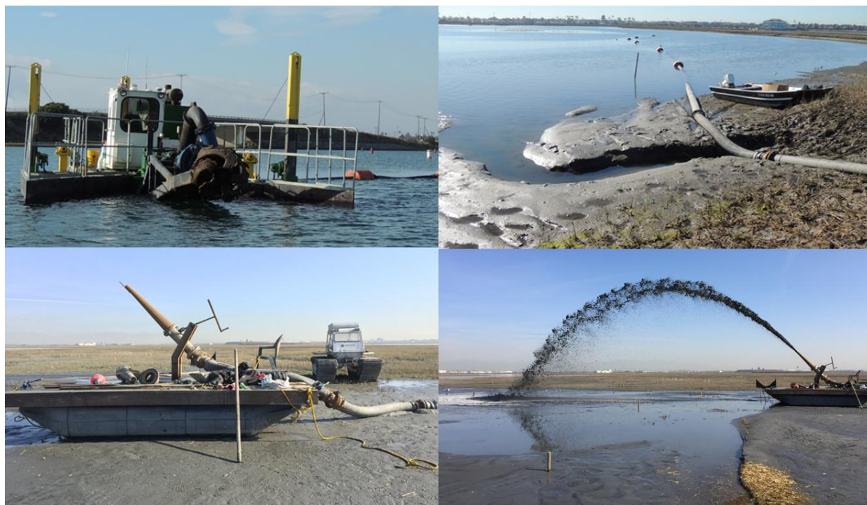
FIGURE 13. THIN LAYER SEDIMENT DEPOSITION CONSTRUCTION METHODS
