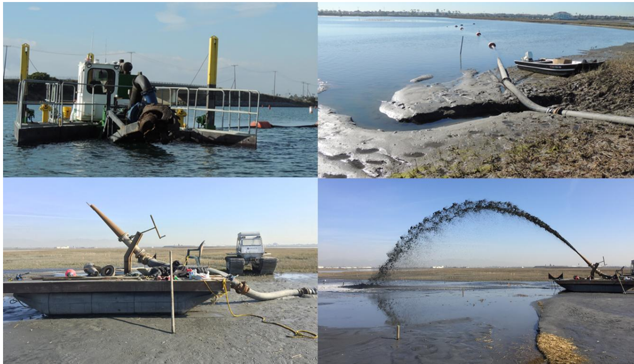
FIGURE 13. THIN LAYER SEDIMENT DEPOSITION CONSTRUCTION METHODS
