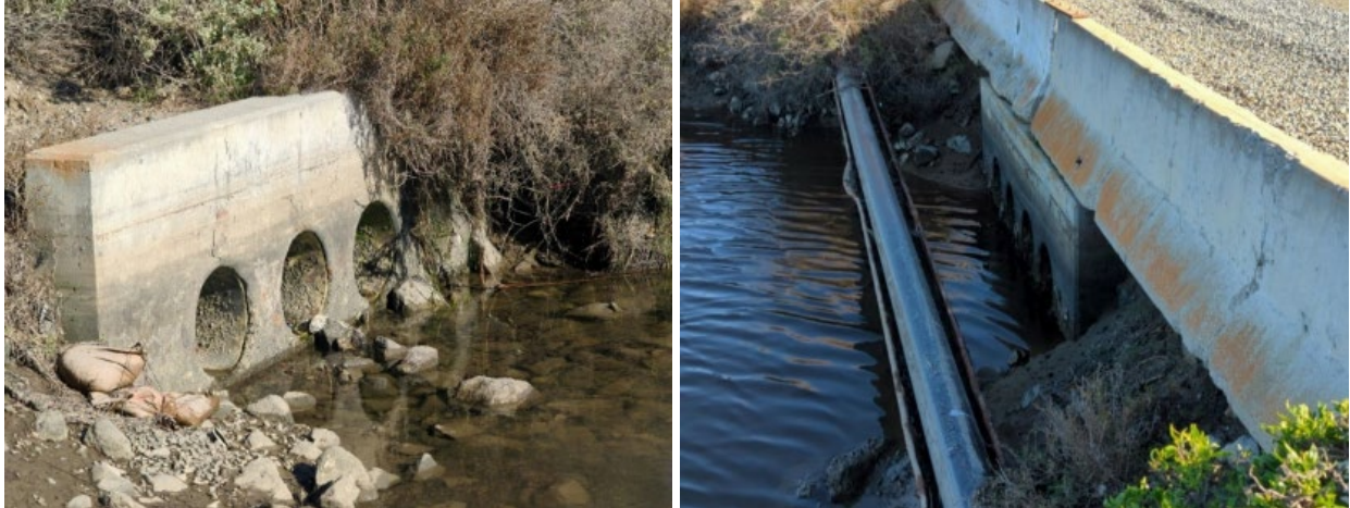
FIGURE 7: CULVERTS UNDER DIRT ACCESS ROADS (USACE 2024)
