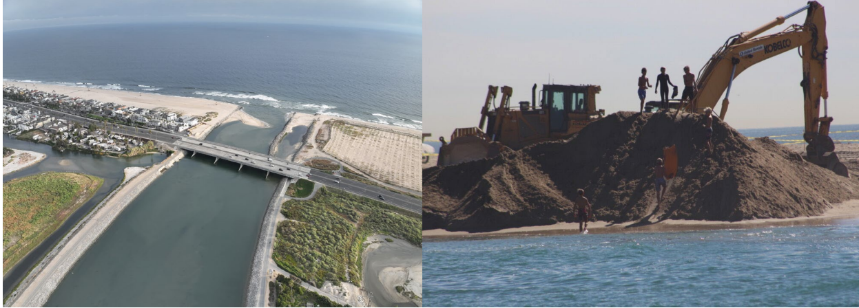
FIGURE 13: SANTA ANA RIVER MOUTH DREDGING
